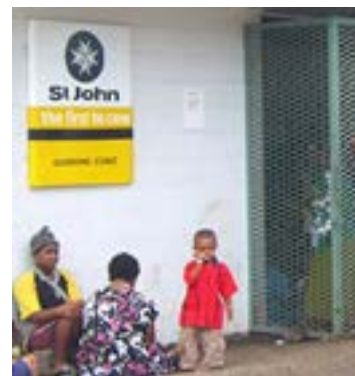
The renovated Gordons Clinic, reopened by St John PNG after being closed for 11 years.
